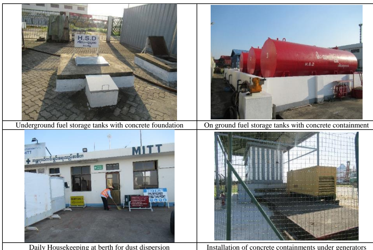
Figure 5.3-7 Photos of mitigation measures for soil contamination
